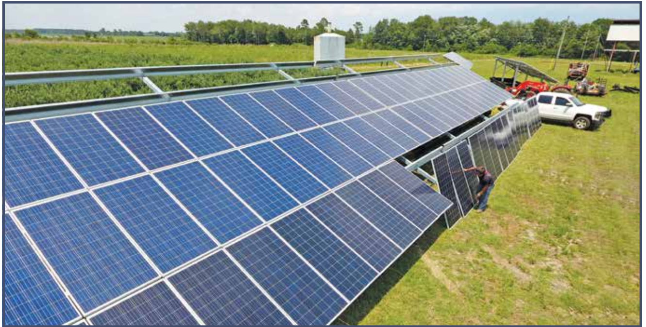
Installation of a 53.76kW solar array at a peanut buying point in Alma. (Photos courtesy Sunbelt Power Solutions)
