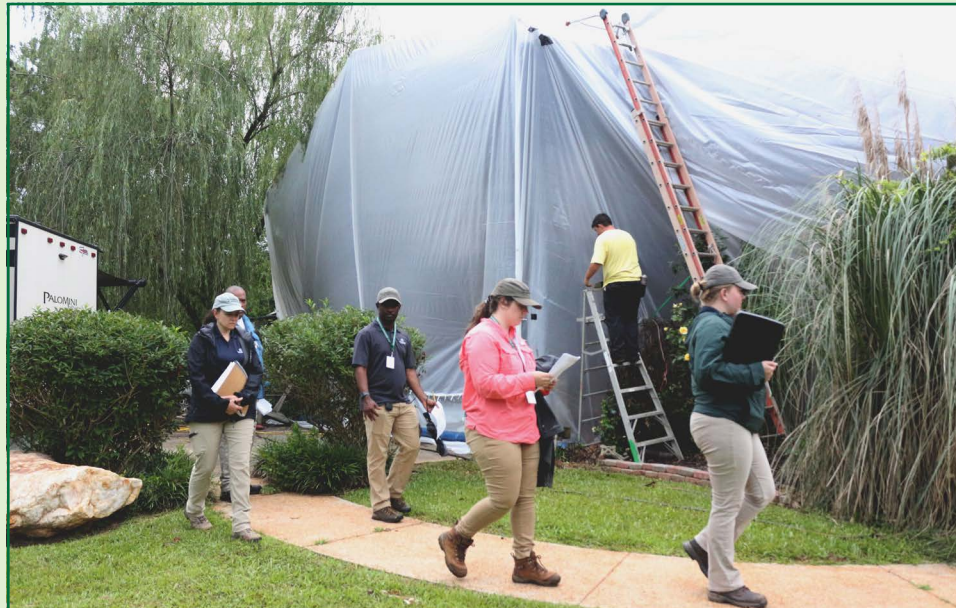
Fumigating a structure requires tenting it with plastic tarps that are taped and clipped together. The Whitesburg structure represented 140,000 cubic feet of living space created by numerous additions to the main structure. Barnes Lakeside Exterminating spent five days wrapping the building prior to fumigating for wood-boring powder post beetles.
