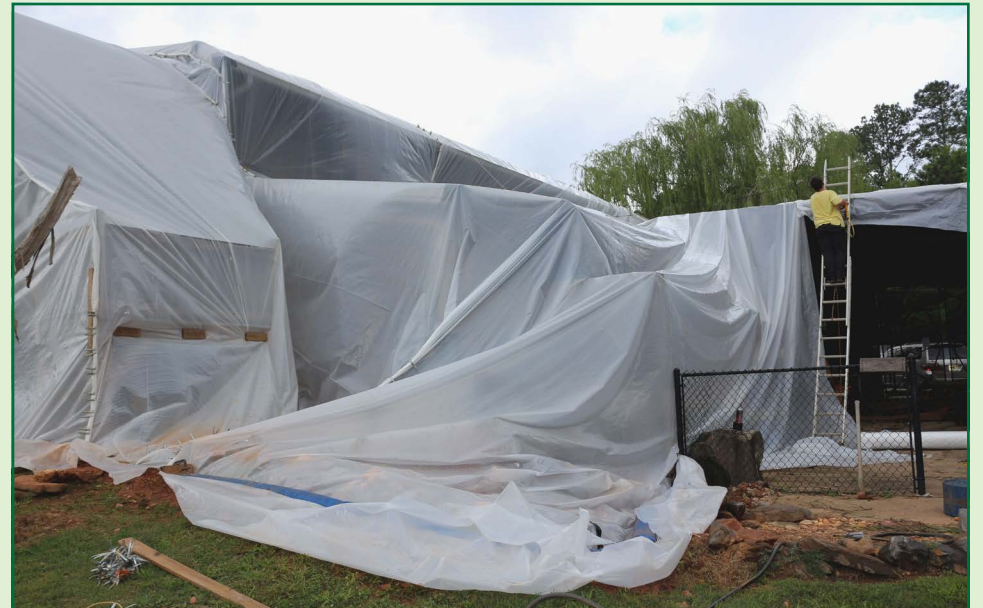
Fumigating a structure requires tenting it with plastic tarps that are taped and clipped together. The Whitesburg structure represented 140,000 cubic feet of living space created by numerous additions to the main structure. Barnes Lakeside Exterminating spent five days wrapping the building prior to fumigating for wood-boring powder post beetles.
