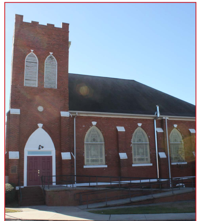
First African Baptist Church on Telfair Street was established in 1867 and is the oldest African American church in Dublin. The current building was built in 1914 after the original wooden church was torn down. A sculpture by local artist, Juan Lleras, stands at the church entrance, calling to new generations to carry on King's legacy of peaceable activism. (GDA/Lee Lancaster)
